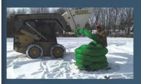
If you're looking for a good BMP for use in cold environments, ice, and snow, check out Filtrexx Siltsoxx. This filtration device is heavy enough to be installed without trenching – great for facilities with frozen ground. Plus, BMP Outlet has a bunch in stock, in case you need to do some last-minute Christmas shopping.
